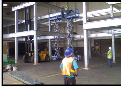
Mezzanine Installation
