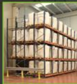
High Density Rack Solutions
