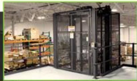
Mezzanine with Freight Elevator
