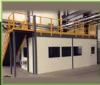
Mezzanine over Modular Building
