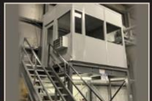
Mezzanine with Modular Building
